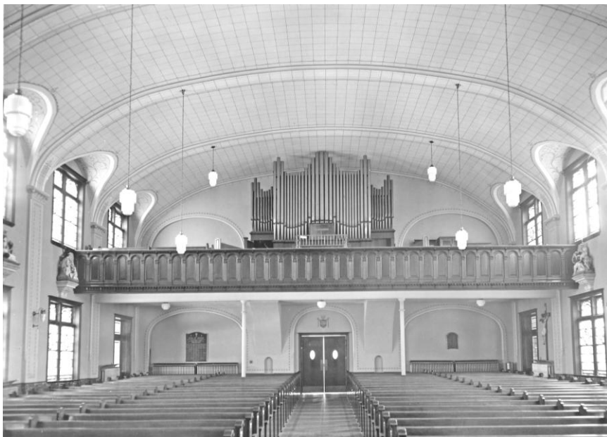
Looking toward back of church after 1943 renovation.
