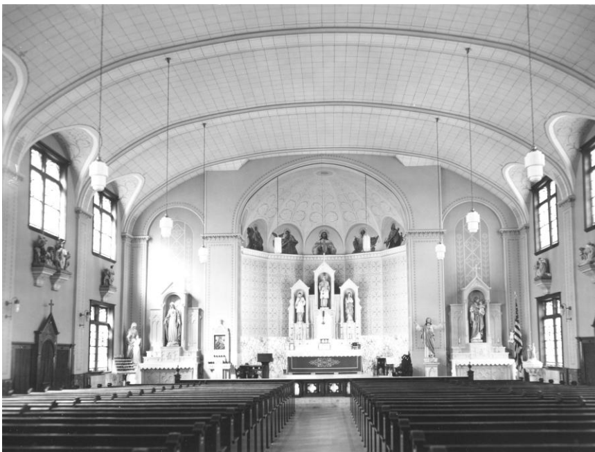
Looking toward the altar after 1943 renovation.
