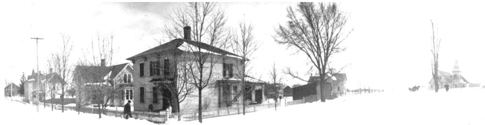
The large house nearest the camera, on the corner of State street and what is now N. Perkins boulevard, was where Mrs. Elizabeth Kennedy hosted an ice cream social fundraiser for St. Charles in 1910. At far right is St. John the Divine Episcopal church.
